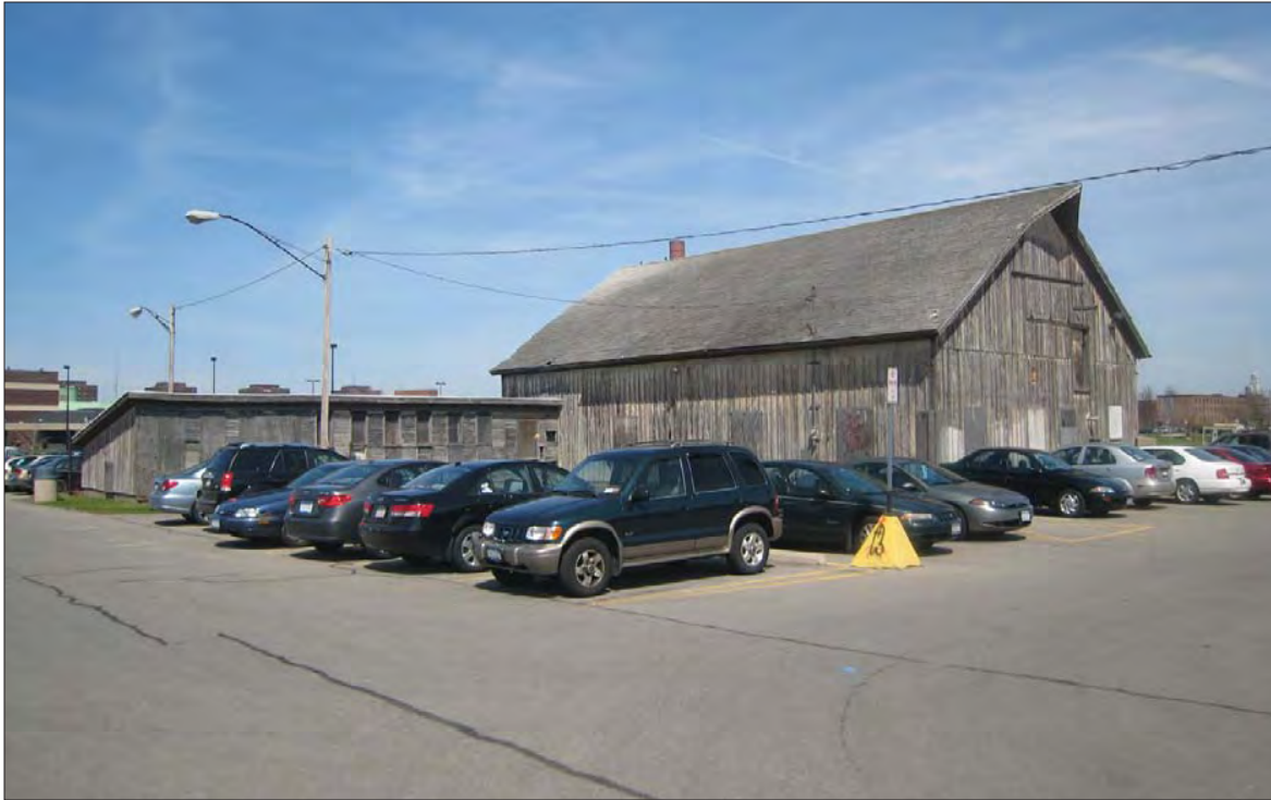
Figure IV.16. View of asphalt parking lot constructed surrounding the former asylum historic wagon shed. Courtesy HL. (R- BRO-2008-04-17-0327.jpg)
