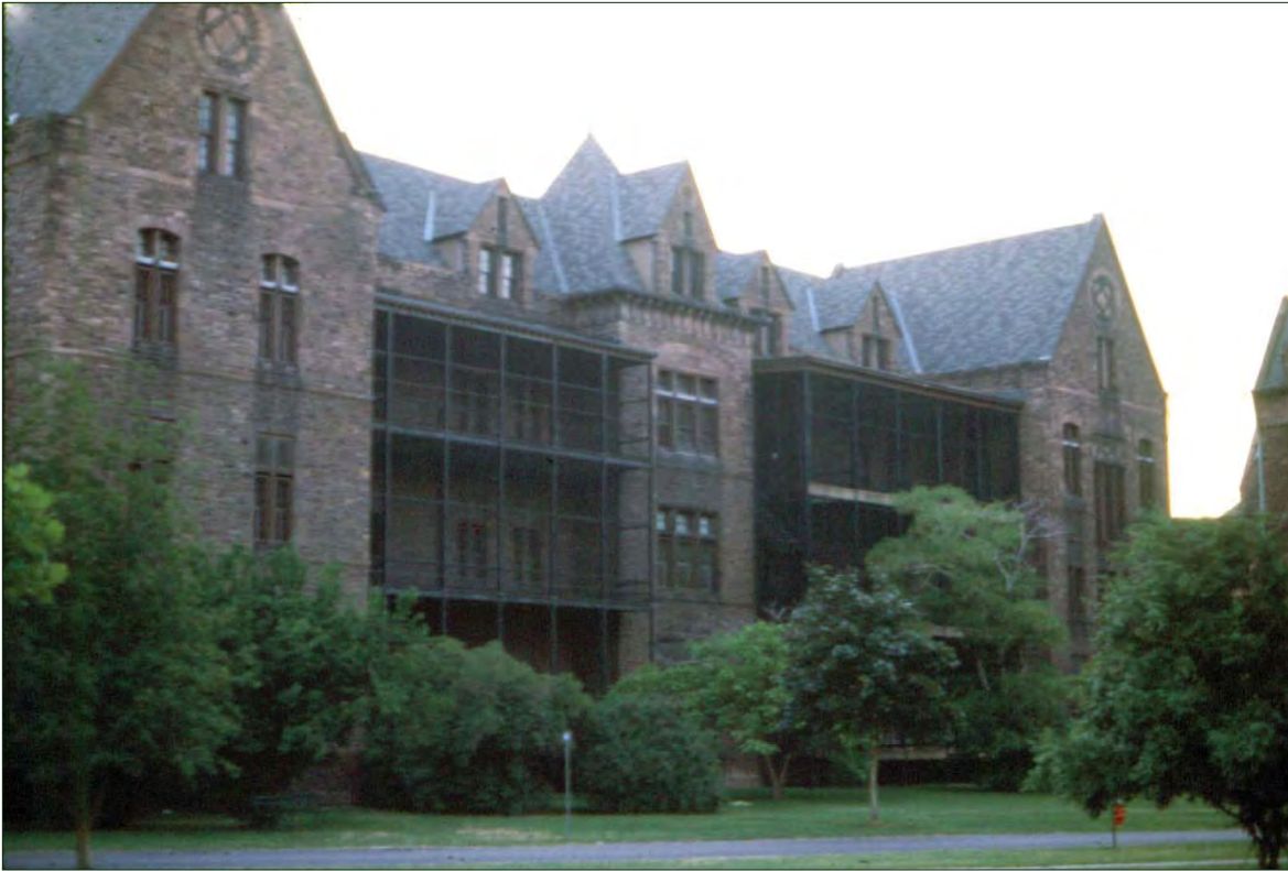
Figure III.52. View of a ward, June 1979. Image courtesy HL. (R-BRO-POD-PatientWard-Veg-1979.jpg)
