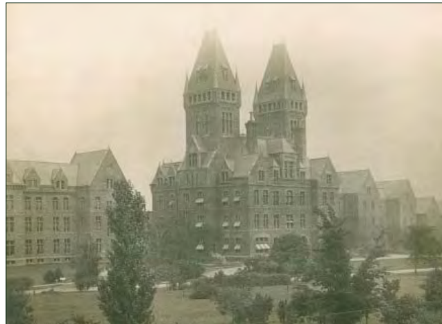
Figure III.21. View looking toward the central Administration Building, c.1895. Improvements to vegetation enhanced the park-like landscape character. Image courtesy Buffalo & Erie County Historical Society. (R-BRO-BHS-2a.jpg)
