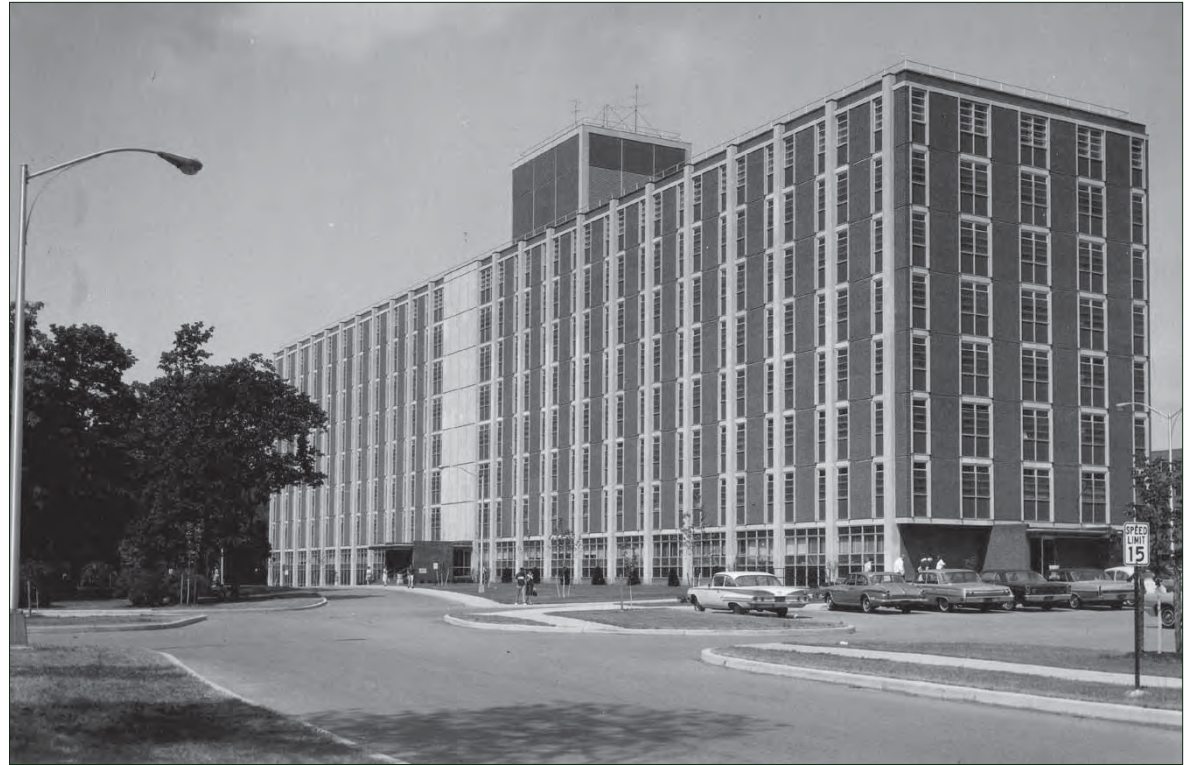
Figure III.48. View of the Strozzi Building. The patient facilities constructed during this period decreased the open space available for patient recreation. Image Courtesy Buffalo Psychiatric Center. (R-BRO-GCA1-Strozzi c196421.jpg)
