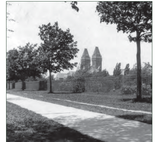
Figure III.22. View looking into the asylum grounds from Forest Avenue. A double row of street tree plantings and the iron perimeter fence define the property edge. Image Courtesy Buffalo Psychiatric Center. (R-BRO-GCA1-admin 10.jpg)
