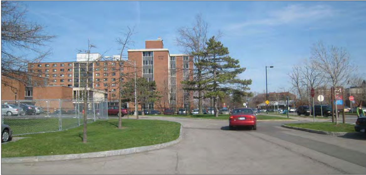
Figure IV.13. The northern area of Landscape Unit 4 once functioned as part of the asylum service area. Today the landscape character and features have little cohesion with the broader asylum landscape. Courtesy HL. (R- BRO-2008-04-17-0419.jpg)
