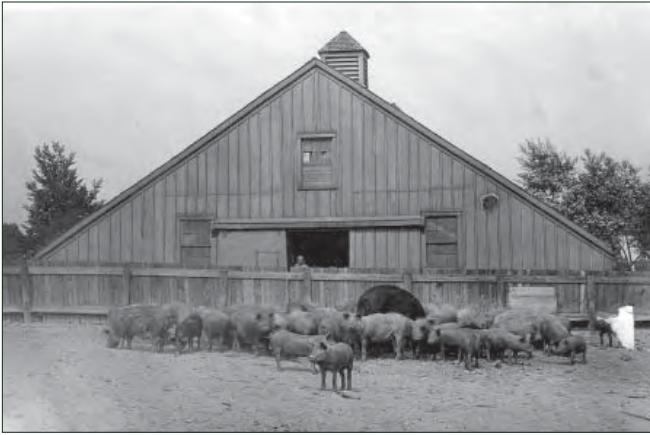
Figure III.17. View of the hog house and wood board fence that enclosed areas for livestock. Image Courtesy Buffalo Psychiatric Center. (R-BRO-GCA1-barn-pigs.jpg)
