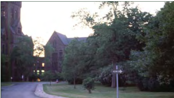
Figure III.53. View of Administration Building and male ward building, June 1979. Image courtesy HL. (R-BRO-POD-Towers-Drive-Veg-1979.jpg)
