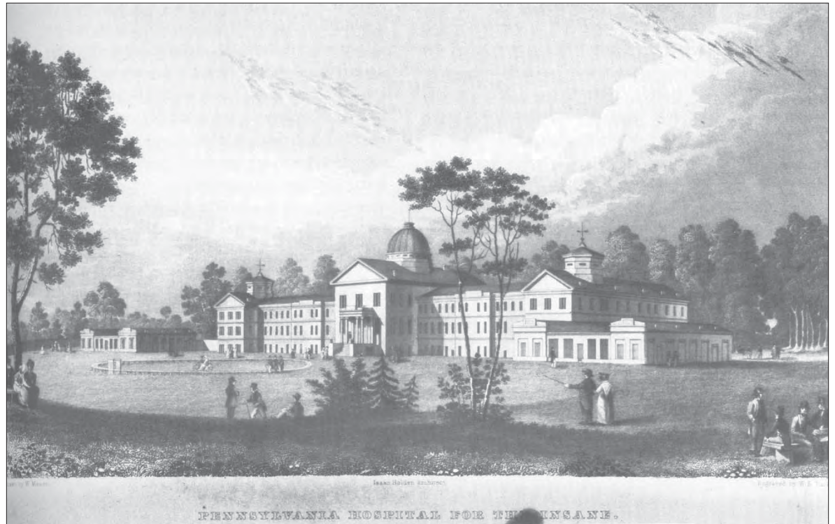
Figure II.5. “ Pennsylvania Hospital for the Insane, Isaac Holden, Architect ” was the first insane asylum building to exemplify Kirkbride's theories. Image reproduced from Yanni, 2007, 39. (R-BRO-PennHospital-Yanni.jpg)
