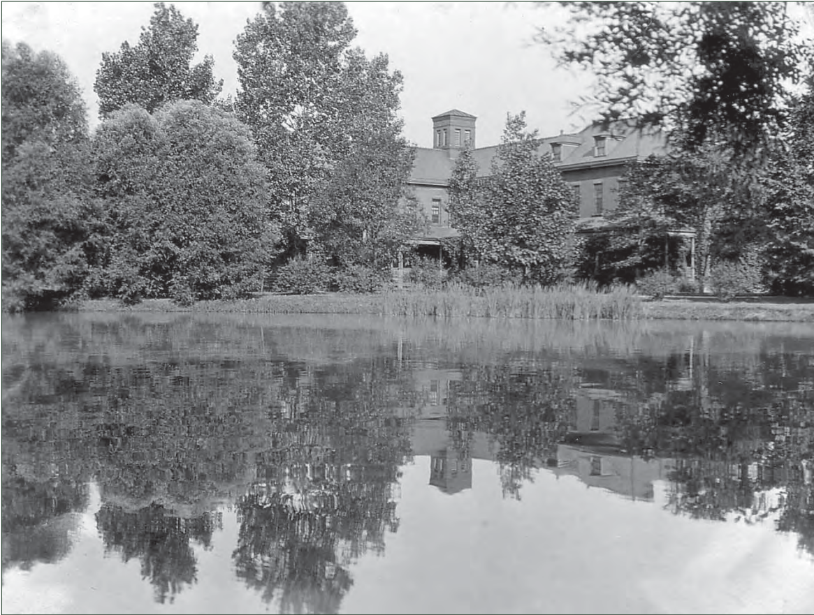
Figure III.29. View looking across the constructed pond to the Elmwood Complex. Dense tree and shrub plantings surrounding the pond and the new patient facilities added to the overall scenic character of the Buffalo State Hospital landscape. Image Courtesy Buffalo Psychiatric Center. (R-BRO-GCA1-bldg & pond.jpg)
