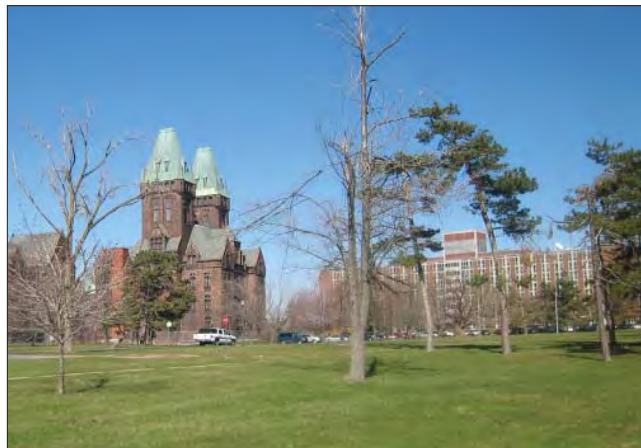
Figure IV.9. View of the towers of the Administration Building. The towers remain visually dominant in the currently fragmented historic landscape. Courtesy HL. (R- BRO-2008-04-16_0122.jpg)
