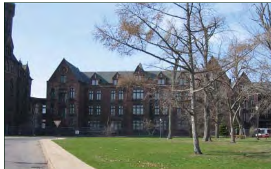
Figure III.54. Contemporary view identical to Figure III.52, April 2008. Image courtesy HL. (R-BRO-20080417_1551.jpg)
