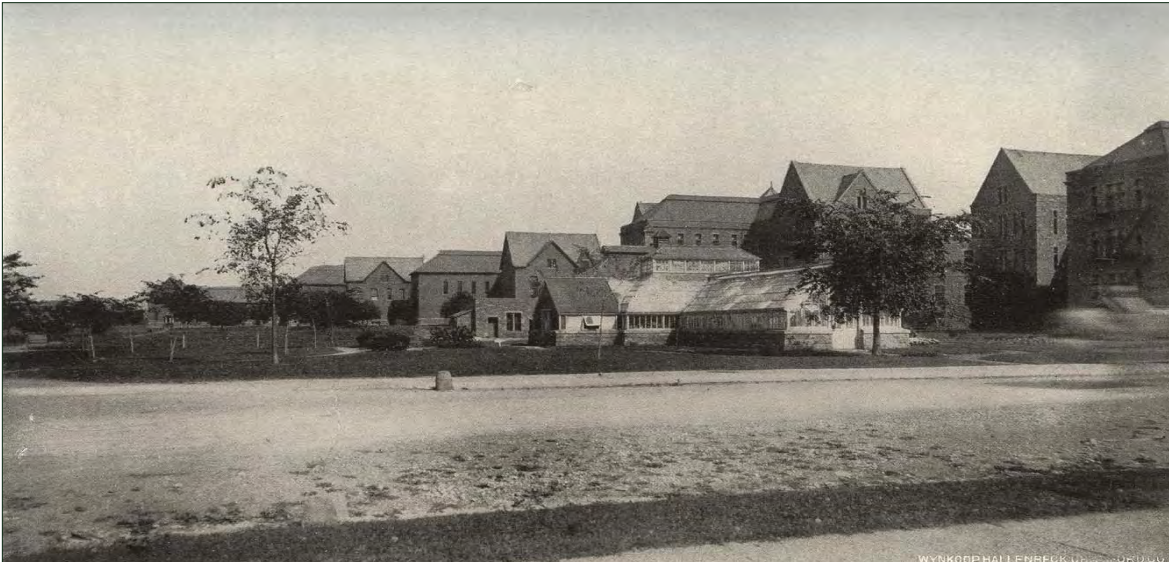
Figure III.24. View looking east toward the greenhouse with the male ward buildings in the background. Nearby drives and walks provided access to the patient recreational facility. Image courtesy Buffalo & Erie County Public Library. (R-BRO-BSAI-AR-Greenhouse-Drive-1897.jpg)
