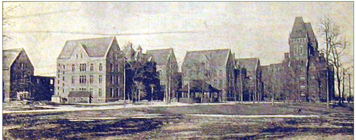
Figure III.26. View looking east toward the female ward buildings. A summerhouse is visible near the center of the image. Nearby trees provided additional shade for the open-air structure. Image courtesy Buffalo & Erie County Public Library. (R-BRO-BEC-FemaleWard-Pavilion-1895.jpg)
