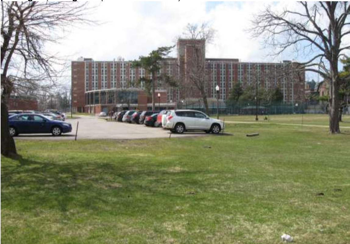
Photograph 12. The eastern and central parts of Study Area C showing an existing parking lot, facing west ( Panamerican 2011 ).
