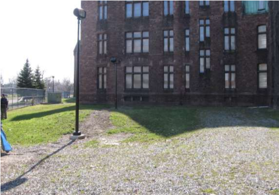
Photograph 5. Gravel and utilities common along the south side of the historic buildings (Buildings #10, #44, #45) facing west-southwest ( Panamerican 2011 ).
