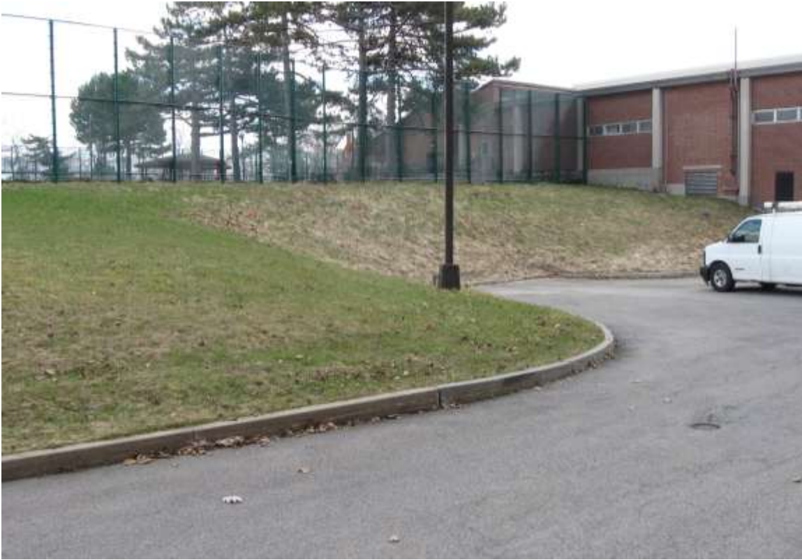
Photograph 9. Grading in the southwestern part of Study Area B, facing southeast (Panamerican 2011).
