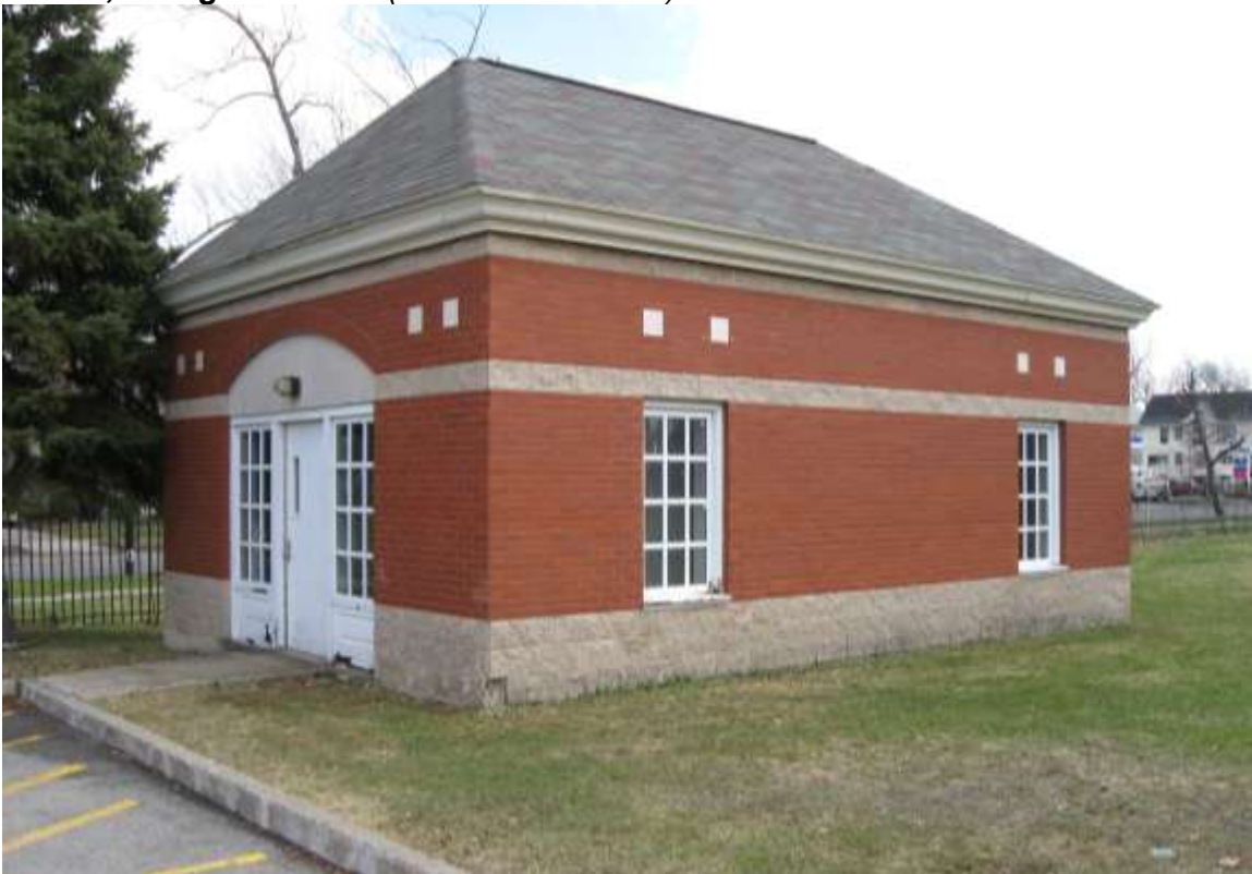
Photograph 14. A modern utility building (c. 1991 valve house [Building 47]) on the east side of Study Area C, facing southeast ( Panamerican 2011 ).
