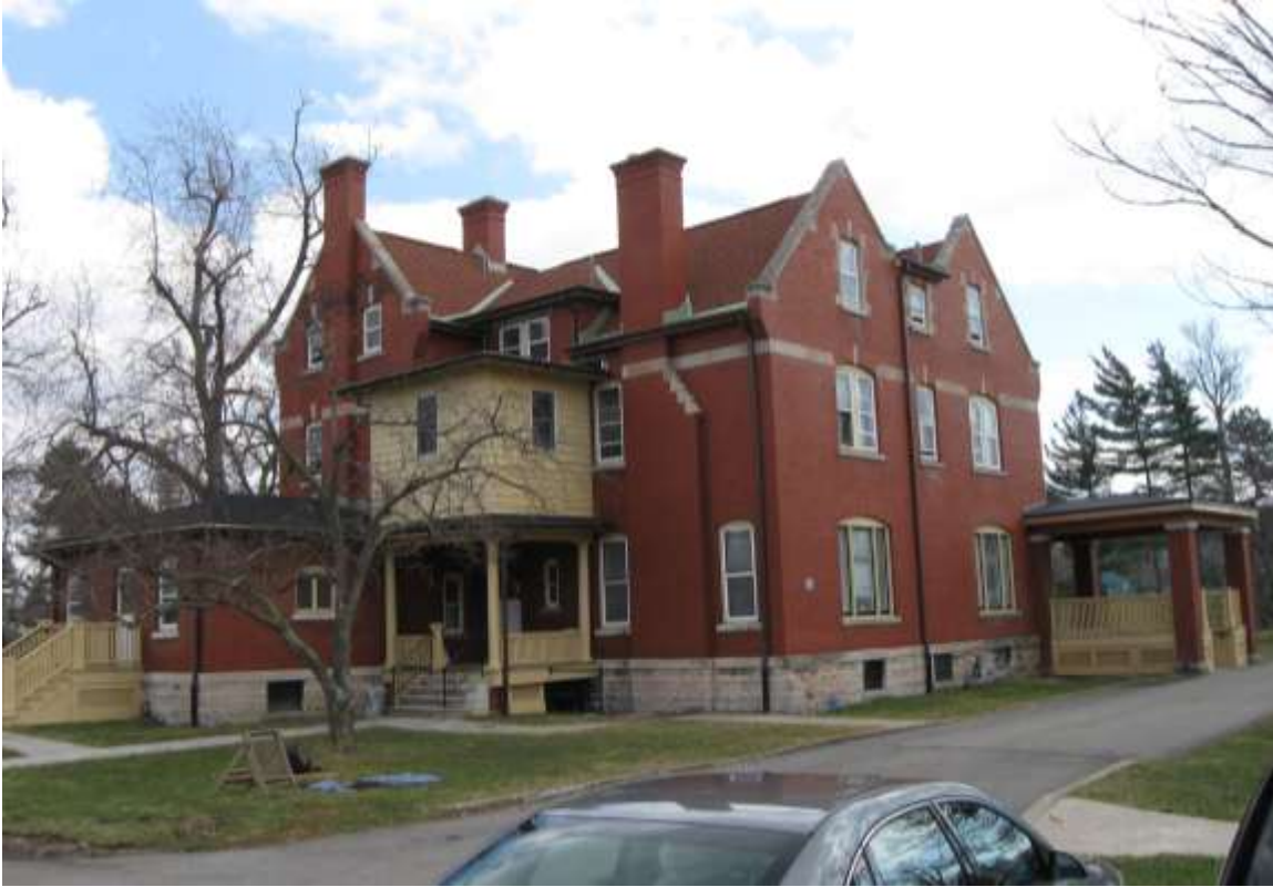
Photograph 13. Rear elevation of Building #1 (c.1912) located just south of Study Area C, facing southeast ( Panamerican 2011 ).
