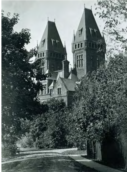
Historic framed view of Building 45
