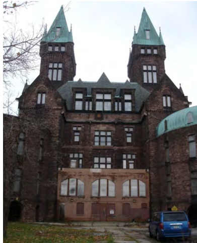
1927 rear addition to Building 45
