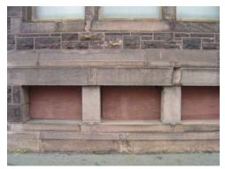
Fig. AB.26 **Stone surface and unit spalling** Image courtesy GCA
