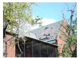
Fig. I.3 **Original slate roof and copper flashings** Image courtesy GCA
