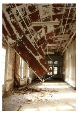
Fig B.64 Severe ceiling damage in Female Ward F  $\ensuremath{\mathsf{Image}}$  courtesy GCA
