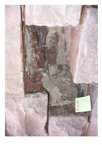
Exploratory Opening EWO-06 in stone masonry wall of Building G.
