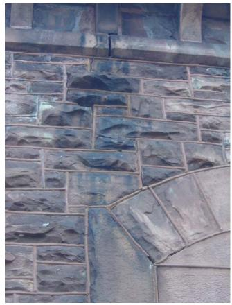
Fig. MK.5 **Step cracking on west elevation** Image courtesy GCA
