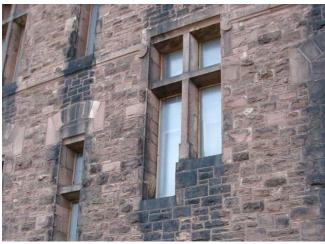
Fig. B.4 Carved scrolled ends where the beltcourse meets the window opening Image courtesy GCA
