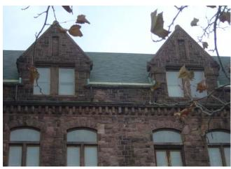
Fig. F.4 Decorative scroll carvings and blind niches at dormer, and rough hewn stone cornice modillions Image courtesy GCA
