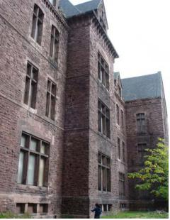
Fig. A. 8 South elevation – iron porch removal, original mortar and patching Image courtesy GCA
