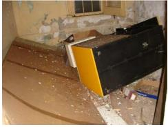
Fig. J.II **Partially collapsed floor in west end** Image courtesy GCA
