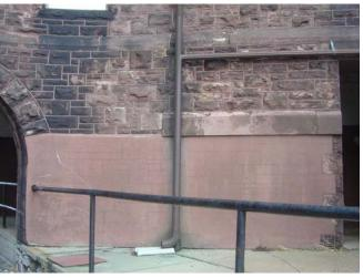
Fig. AB-F.3 **Crack at junction with main building** Image courtesy GCA
