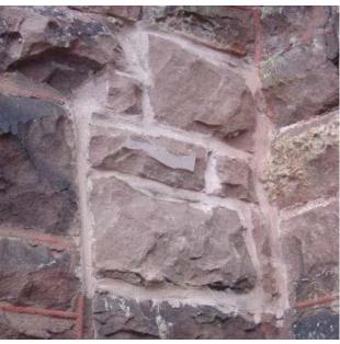
Fig. AB.2I **Stone infill at beam locations** Image courtesy GCA
