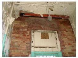
Fig. G.10 Typical interior condition at ongoing water infiltration locations Image courtesy GCA
