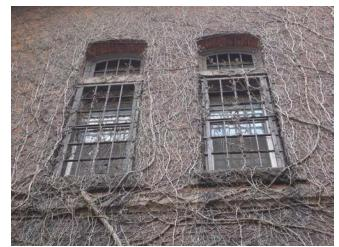
Fig. H.6 **lvy growth on north elevation** Image courtesy GCA
