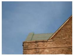
Fig. B.II **Asphalt shingles cover the gable rake** Image courtesy GCA
