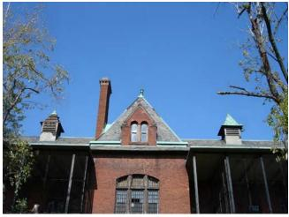
Fig. 1.5 **Photo of ventilation cupolas – current condition** Image courtesy GCA
