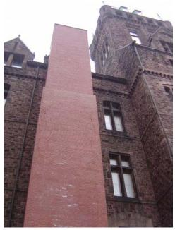
Fig. AB.32 **Brick elevator shaft on west elevation** Image courtesy GCA
