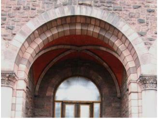
Fig. AB.6 **Brick vaulting at main entrance** Image courtesy GCA
