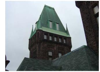
Fig. AB.13 **Copper tower roof** Image courtesy GCA
