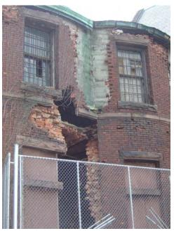
Fig.H-I.3 **Detail of collapse and previous repair** Image courtesy GCA
