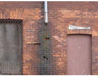
Fig. FK.6 **Typical soiling, spalling and open joints at brick gables** Image courtesy GCA
