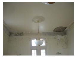
Fig. A.15 **Plaster damage at roof or downspout leak** Image courtesy GCA
