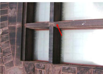
Typical cracking (arrow) of vertical intermediate mullions.
