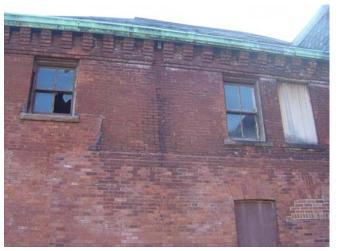
Fig. FK.7 Missing downspout and resulting masonry deterioration Image courtesy GCA
