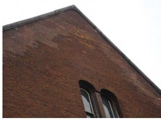
Fig. H.7 Detail of previous repointing and ongoing deterioration of masonry Image courtesy GCA
