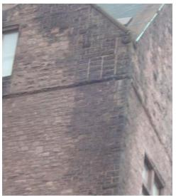
Fig. F.10 Northeast corner – detail of masonry deterioration Image courtesy GCA
