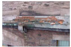
Fig. AB.17 North elevation plywood and stucco cornice Image courtesy GCA
