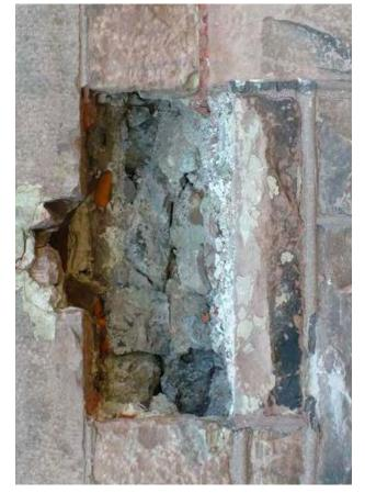
Exploratory Opening EWO-09 in stone masonry wall of Building F.
