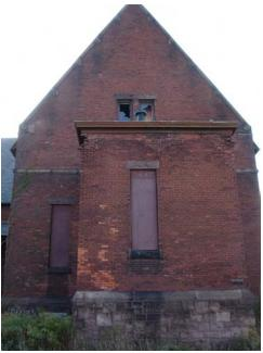
Fig. J.8 East elevation showing areas of collapse and step cracking above attic window Image courtesy GCA
