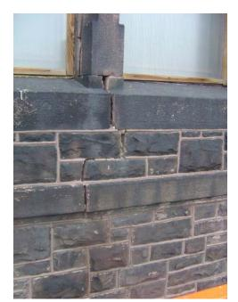
Fig. EX.14 Step crack through mortar joints in stone facade Image courtesy GCA
