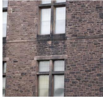
Fig. A.7 **Step cracking on north elevation** Image courtesy GCA
