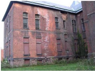
Fig. I.7 Saturated masonry and mortar deterioration Image courtesy GCA
