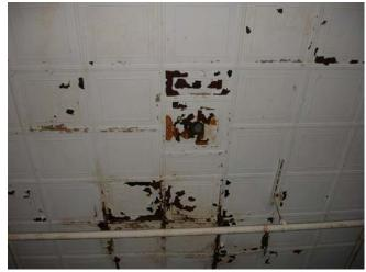
Fig. J.12 Area of water infiltration exposing framing  $\ensuremath{\mathsf{Image}}$  courtesy GCA
