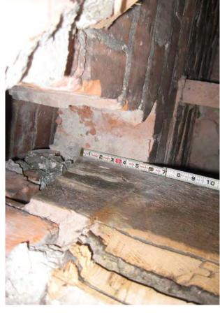
Exploratory Floor/Wall Opening IWO-02 at an exterior wall in Building H. This shows the firecut floor joists.
