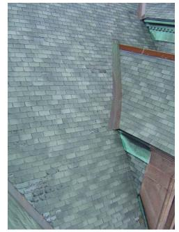
Fig. AB.14 **Asphalt roof - deteriorating condition** Image courtesy GCA
