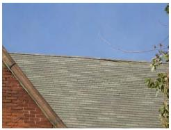
Fig. J.9 **Typical condition of asphalt shingle roof** Image courtesy GCA
