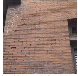
Fig. H.8 **Efflorescence and spalling of brick** Image courtesy GCA
