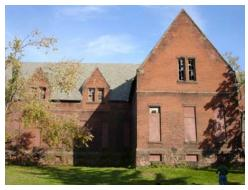
Fig. J.10 South elevation showing plywood coverings on lower windows and broken panes on attic windows
