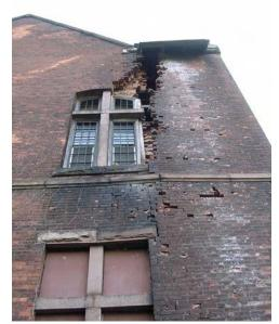
Fig B.60 **Severe water damage in Female Ward H** Image courtesy GCA
