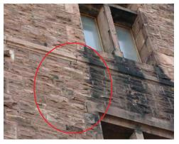
Fig. B.9 **Step cracking on the east elevation** Image courtesy GCA
