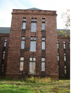
Fig. B.8 Alterations to central north bay for previous fire escape Image courtesy GCA
