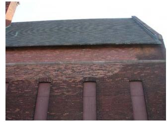
Fig. J.4 Area of previous brick rebuilding on north elevation  $\ensuremath{\mathsf{Image}}$  courtesy GCA
