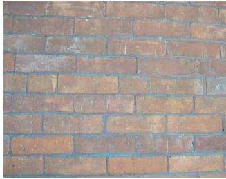
Fig. H.13 **Original red mortar evident at porch area** Image courtesy GCA
