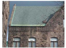
Fig. F.3 **Frieze stones in stack bond** Image courtesy GCA
