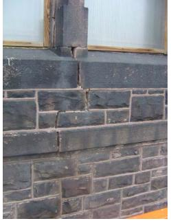
Fig. AB.28 **Step crack through mortar joints** Image courtesy GCA
