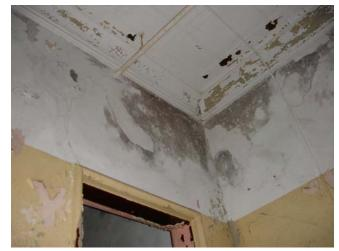
Fig. J.13 **Typical condition of surfaces due to moisture - peeling paint, mold, rusted ceilings** Image courtesy GCA
