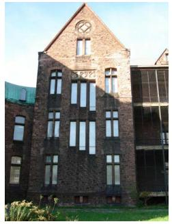
Fig. B.2 Red Medina stone is contrasted with yellow sandstone to create decorative patterns Image courtesy GCA
