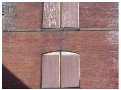
Fig. FDH.3 **Detail of brick jack arch and sandstone beltcourse, keystone, quoins and sill** Image courtesy GCA
