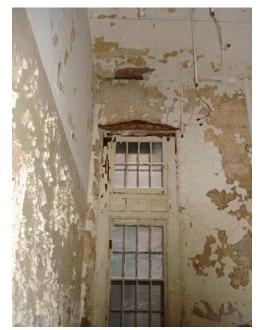
Fig. G.II **Typical interior condition due to high moisture content** Image courtesy GCA
