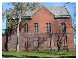
Fig. 1.10 Saturated masonry and mortar failure below gable capstone Image courtesy GCA
