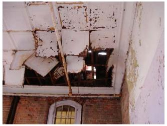
Fig. 1.13 **Rusted tin ceiling and structural damage** Image courtesy GCA
