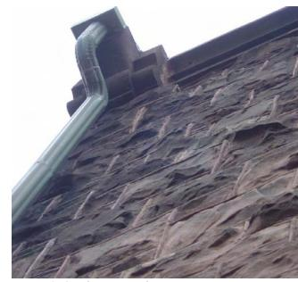
Fig. AB.24 **Shifted (and repaired) cornice stones** Image courtesy GCA
