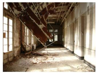
Fig. F.I4 **Rusted, falling tin ceilings** Image courtesy GCA
