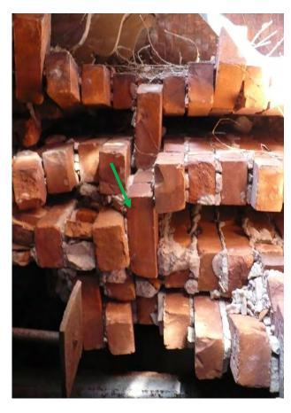
Typical wall construction at brick buildings (photo taken at area of severe damage). Outer two wythes (though the outermost wythe is delaminating from the second wythe in the photo) are tied to the inner two wythes (left side of photo) by header bricks that span the cavity (arrow).
