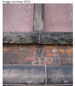
Fig. H.II Step cracking at brick and stone – north elevation Image courtesy GCA
