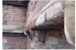
Fig. AB.16 North elevation plywood and stucco cornice
