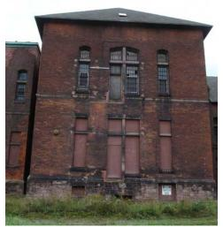
Fig. H.10 Previous alterations for fire escape – north elevation
