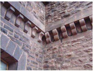
Fig. AB.8 **Cornice brackets** Image courtesy GCA
