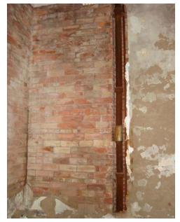
Fig. G.8 Internal downspout and associated plaster and wall damage Image courtesy GCA
