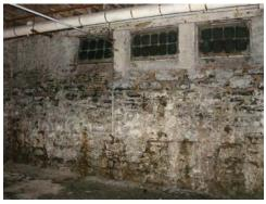
Fig. G.9 Basement water infiltration through wall
