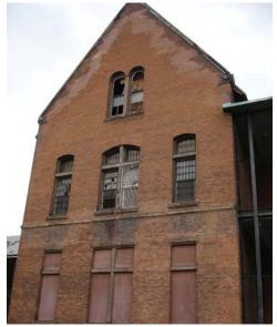
Fig. H.9 Previous repointing and ongoing deterioration Image courtesy GCA
