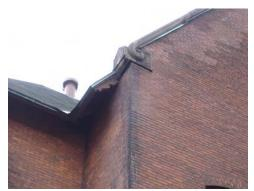
Fig. H.3 Gable cap stone decorative scroll carving and wooden rafter tail detail Image courtesy GCA
