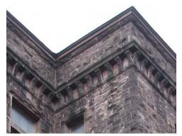
Fig. G.2 North Elevation showing cornice and bracket detail Image courtesy GCA
