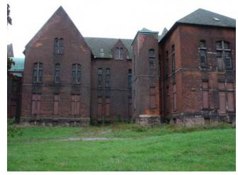
Fig. H.5 Overall elevation showing soiling and spalling at brick wall Image courtesy GCA
