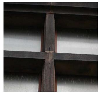
Fig. A.5 **Vertical cracking at stone window muntin** Image courtesy GCA
