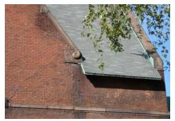
Fig. J.2 Decorative scroll carving at gable cap stone Image courtesy GCA
