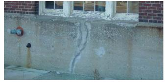
Fig. MDH.4 **Foundation wall crack on east elevation** Image courtesy GCA
