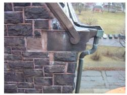
Fig. AB.25 **Shifted (and repaired) cornice stones** Image courtesy GCA
