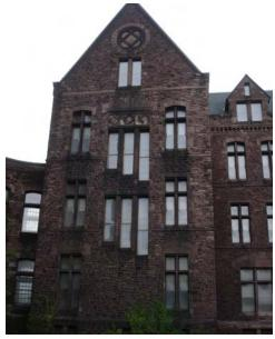
Fig. A.2 South elevation showing decorative features – cornice modillions and brackets, and windows in dormer gable peaks Image courtesy GCA
