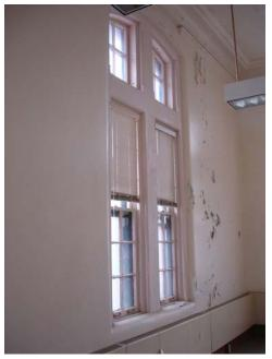
Fig. A.16 **Moisture damage to walls** Image courtesy GCA
