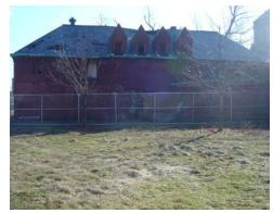
Fig. FK.3 Female Kitchen West Elevation showing sagging roof ridge Image courtesy GCA
