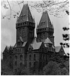
Fig. AB.10 Historic photo showing original clay tile on towner and slate roof on main building Image courtesy GCA
