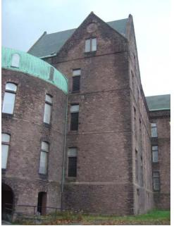
Fig. F.8 Northeast corner showing saturation of masonry below gable and at corner (dark stone) Image courtesy GCA
