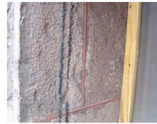
Fig. AB.30 **Original mortar at window jambs** Image courtesy GCA
