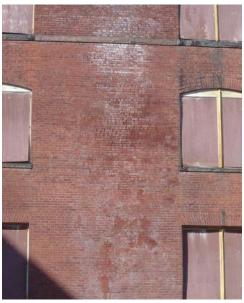
Fig. FDH.4 Area of water saturation showing mortar erosion and efflorescence Image courtesy GCA
