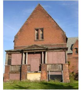
Fig. J.5 West wall of north wing with wooden porch - area of bulging and previous stabilization efforts
