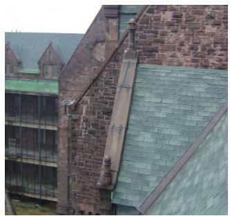
Fig. AB.23 **Iron cramps at dormer gable rake stones** Image courtesy GCA
