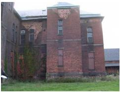
Fig. 1.9 Brick failure at north elevation Image courtesy GCA
