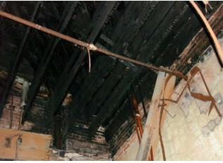
Fig. G.12 Fire damage to Room 10 Image courtesy GCA
