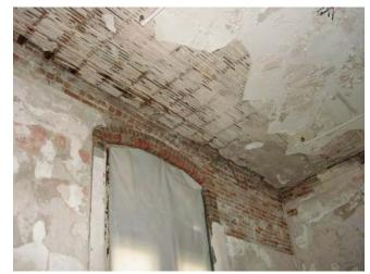
Fig. B.13 **Plaster damage at walls and ceiling** Image courtesy GCA
