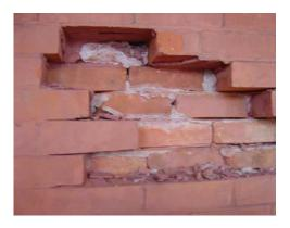
Fig IN.4 **Exploratory probe in brick wall** Image courtesy GCA
