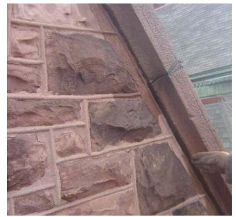
Fig. AB.22 Lifted and displaced gable stones Image courtesy GCA
