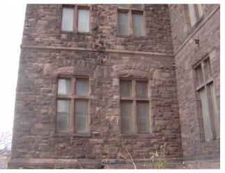
Fig. F.7 South elevation – stone conditions at removed west porch  $\mathsf{Image}\xspace$  courtesy GCA
