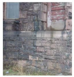
Fig. F-G.3 North elevation door opening, step crack below Image courtesy GCA
