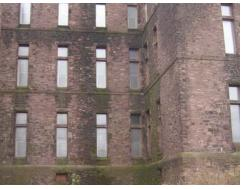
Fig. F.9 Elevation showing algae (green), soiling (black), and spalled areas (light red) Image courtesy GCA
