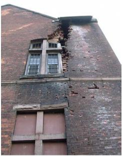
Fig. 1.8 **Brick failure at north elevation** Image courtesy GCA
