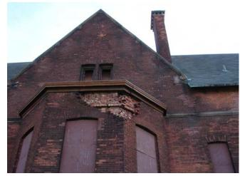
Fig. J.3 **Areas of brick collapse on north elevation** Image courtesy GCA
