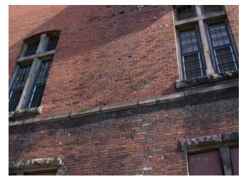
Fig. 1.6 Surface conditions of brick showing spalling, efflorescence and soiling Image courtesy GCA
