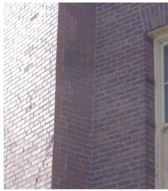
Fig. MDH.3 **Area of corner rebuilding** Image courtesy GCA
