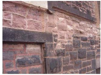
Fig. AB.29 Original mortar exposed where north elevation enclosure removed
