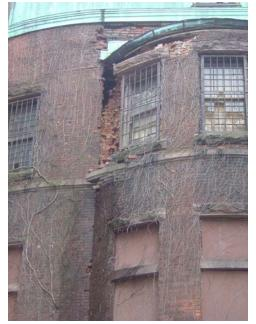
Fig.G-H.3 **Collapsed brick at curved bay to connector** Image courtesy GCA
