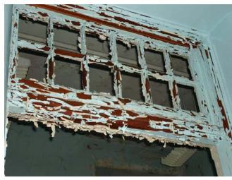
Fig. B.12 **Peeling paint at door and window trim** Image courtesy GCA
