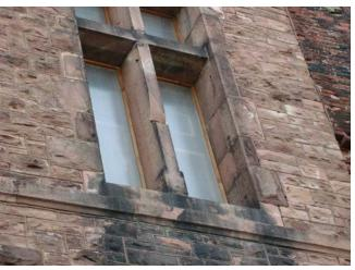
Fig. B.7 **Spalled stone due to embedded rusting iron fasteners** Image courtesy GCA
