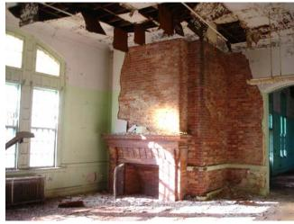
Fig. 1.12 Surface finish damage - missing plaster exposing brick, rusted tin ceiling - at fireplace Image courtesy GCA
