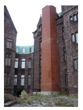
Fig. T.I Incompatible elevator addition on west facade of Administration Building Image courtesy GCA
