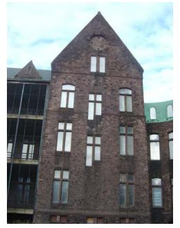
Fig. F.2 Low relieving arches with diamond pattern carvings and gable peak carving Image courtesy GCA
