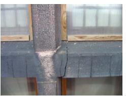
Fig. AB.27 Crack through stone with displacement
