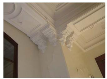
Fig. AB.35 **Decorative plaster brackets and moldings** Image courtesy GCA
