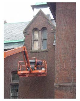
Fig IN.3 Aerial lift survey being undertaken by GCA & SGH team Image courtesy GCA
