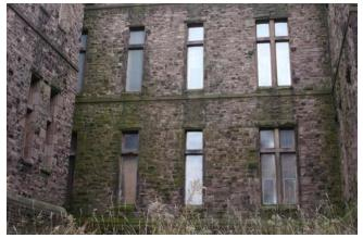
Fig. G.5 **North Elevation showing algal growth** Image courtesy GCA
