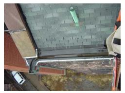
Fig. AB.II Stone scupper, downspout and copper gutter coated with plastic membrane Image courtesy GCA
