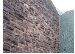
Fig. AB.31 **Typical mortar joint condition** Image courtesy GCA
