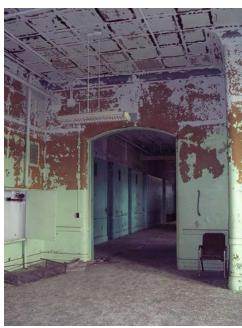
Fig. H.15 Surface finish damage - peeling paint and rusted tin ceilings Image courtesy GCA
