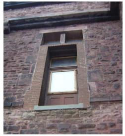
Fig. AB.20 Window opening modified to door opening Image courtesy GCA
