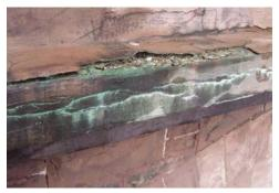
Fig. AB.18 North elevation plywood and stucco cornice Image courtesy GCA
