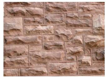
Fig. B.6 Example of red mortar used in some repointing campaigns Image courtesy GCA
