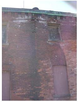
Fig. FK.5 **Brick displacement at cornice and wall** Image courtesy GCA
