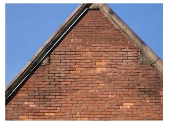
Fig. J.6 Typical soiling, spalling and open joints at brick gables  $\mathsf{Image}\xspace$  courtesy GCA
