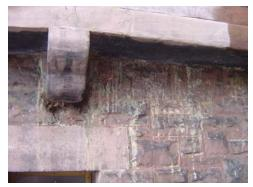
Fig. AB.19 Bird or bat droppings below plywood/ stucco cornice Image courtesy GCA
