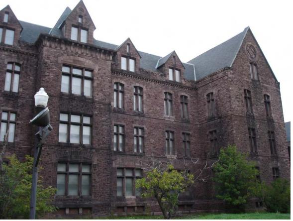
Fig. A.I South elevation overview showing decorative features - contrasting yellow and red sandstone in gable and carved scrolled beltcourse ends Image courtesy GCA
