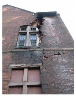
Fig. EX.I5 Brick failure at north elevation in Female Ward I Image courtesy GCA
