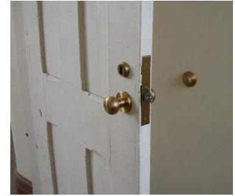
Fig. A.13 **Restored door with retrofit hardware** Image courtesy GCA
