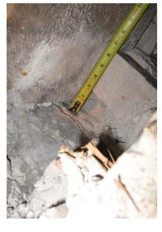
Exploratory Floor/Wall Opening IWO-01 in the third floor of Building B. The floor joists are bearing approximately 5-1/4 in. on the masonry below.
