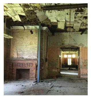
Fig. 3-27: Stabilization in room 30, first floor (CJSA 2019)
