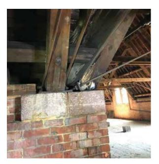
Fig. 3-44: Damaged roof structure (SGH 2019)
