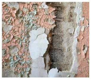
Fig. 3-13: Detail of downspout damage (CJSA 2019)
