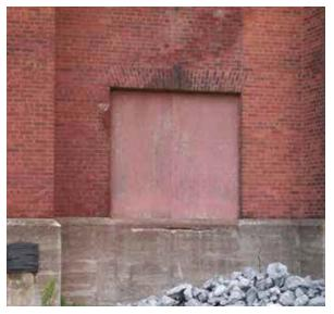
Fig. 3-48: West elevation, water infiltration and crack in concrete (CJSA 2019)
