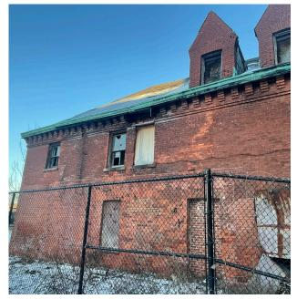
West Elevation Roof Damage and Deteriorated and Failing Masonry
