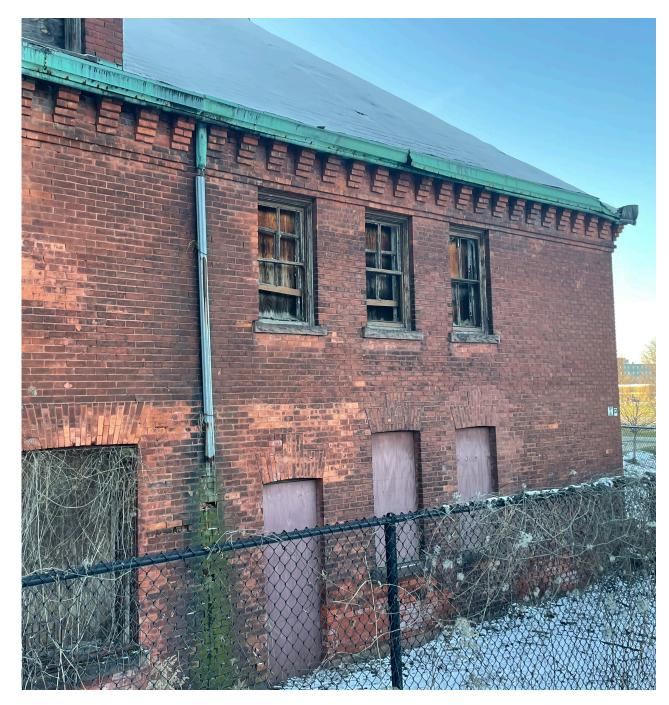
East Elevation Roof Damage and Deteriorated and Failing Masonry. Note Extant Four-Light Wood Sash.
