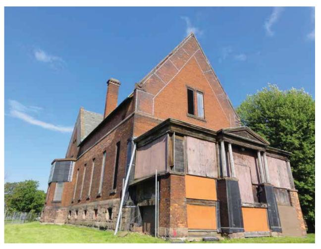
Fig. 3-33: Northwest corner and failing wooden porch (SGH 2019)
