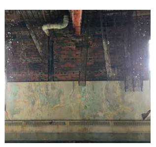
Fig. 3-52: Plaster and ceiling damage on third floor, note exposed structure (CJSA 2019)
