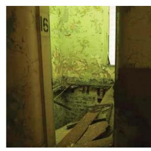
Fig. 3-41: Room 24 with collapsed floor (CJSA 2019)
