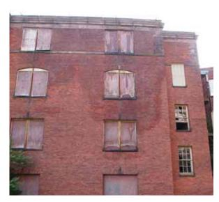
Fig. 3-47: Water infiltration on west elevation (CJSA 2019)
