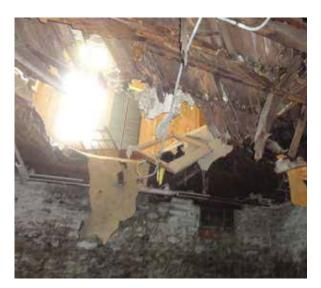
Fig. 3-31: Collapsed portion of first floor (SGH 2019)
