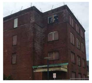
Fig. 3-46: Northeast corner of FDH with standing seam copper shed roof (CJSA 2019)
