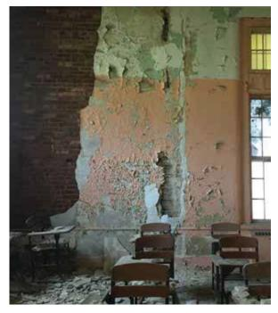
Fig. 3-12: Room 28, First Floor. Typical interior damage from broken downspout (CJSA 2019)
