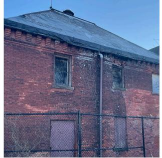
North Elevation Roof Damage and Deteriorated and Failing Masonry
