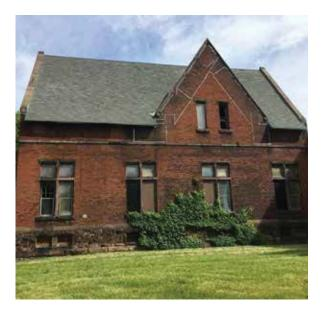
Fig. 3-38: South elevation showing replacement asphalt roof (CJSA 2019)
