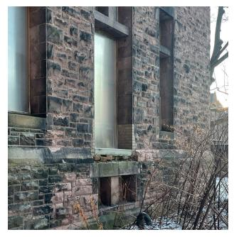
Detail of Deterioration of Mortar Joints
