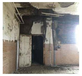
Fig. 3-51: Ceiling damage in Room 6, northwest corner of the third floor (CJSA 2019)
