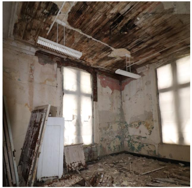
Deteriorated Ceiling Plaster on Third Floor
