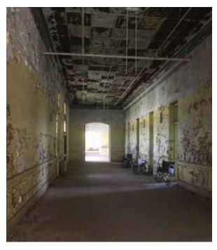
Fig. 3-11: Room 129, First Floor. Typical interior finish conditions in hallway (CJSA 2019)
