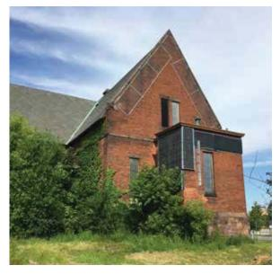
Fig. 3-34: Northeast corner with metal netting stabilization (CJSA 2019)
