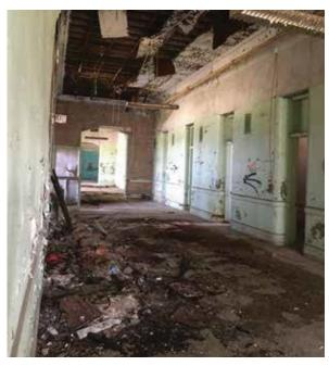
Fig. 3-29: Floor and ceiling damage, second floor hallway looking west (CJSA 2019)
