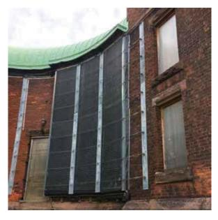
Fig. 3-69: Wall bracing, South Elevation (CJSA 2019).
