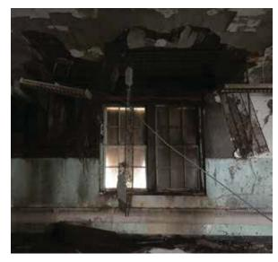
Fig. 3-50: Third floor ceiling and wall damage, looking west (CJSA 2019)
