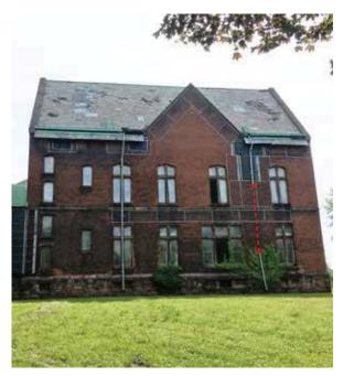
Fig. 3-25: West Elevation, note missing portion of modern downspout (CJSA 2019)
