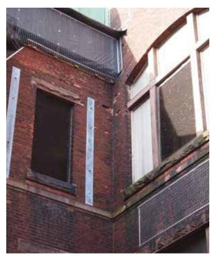
Fig. 3-57: Corner masonry loss (CJSA 2019).
