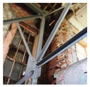
Fig. 3-42: Room 33, masonry damage and stabilization (CJSA 2019)
