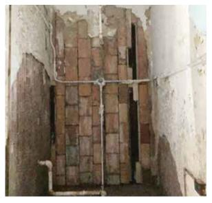
Fig. 3-18: Terra cotta ceiling exposed, second floor (CJSA 2019)
