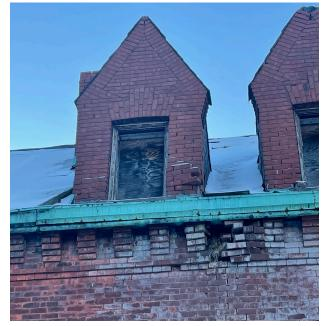
East Elevation Dormer Failing Masonry Detail
