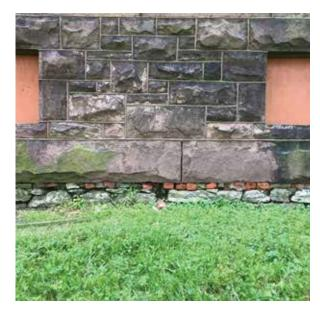
Fig. 3-35: Exposed foundation stones and brick on west elevation (CJSA 2019)
