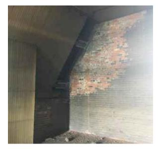
Fig. 3-20: Gable wall damage and stabilization in attic (CJSA 2019)
