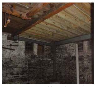
Fig. 3-32: Previous floor stabilization (SGH 2019)
